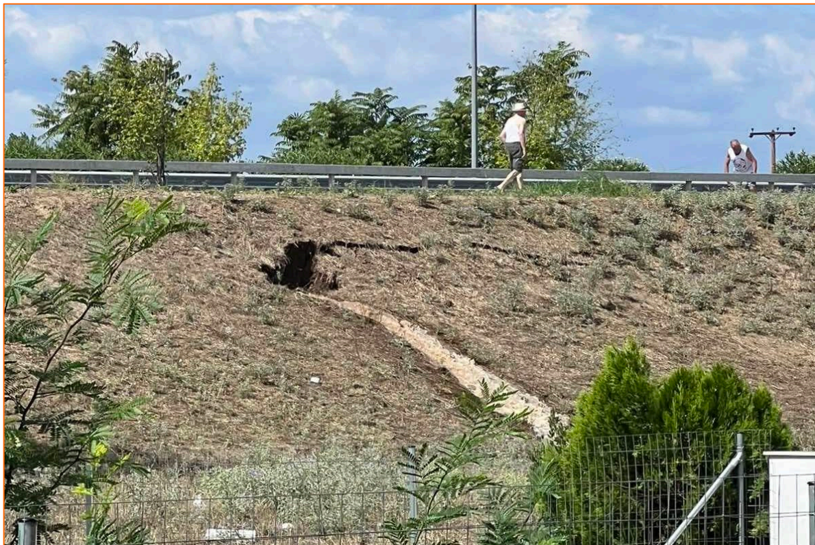
Characteristic views of structural failures of embankment close to Larissa city due to the intense flooding (left) and near Giannouli area (Larissa regional unit; right).
