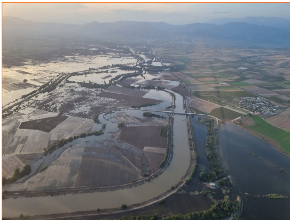
Inundation around Pineios River
