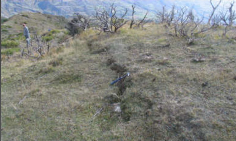
Tension cracks on the ridge crest –potential for landsliding to affect the RoW.
